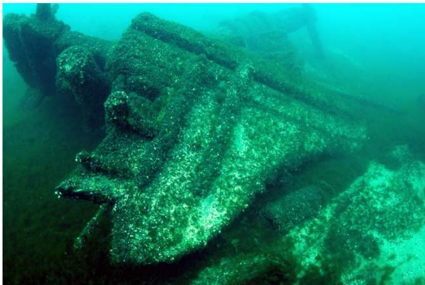
Figure 65. The *Mahoning*'s bow knee. The windlass is visible aft of the stem. Tamara Thomsen.
