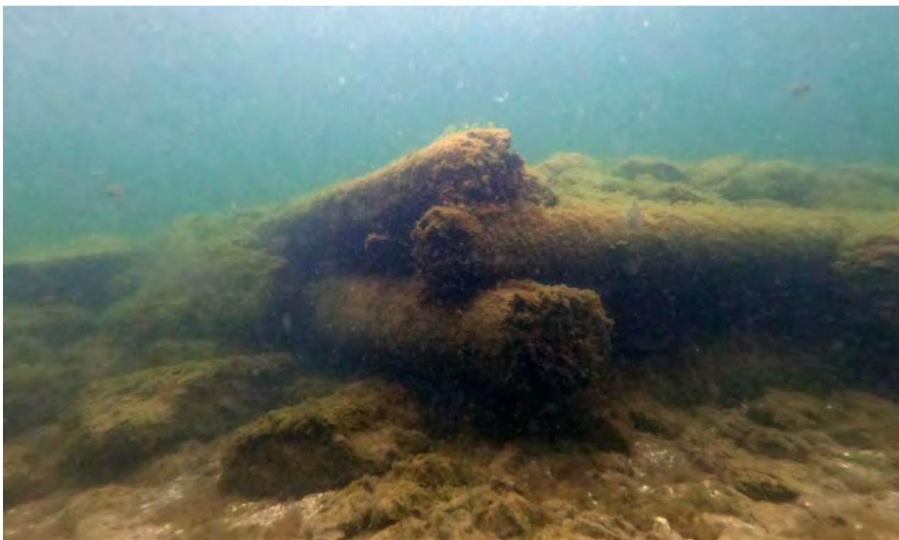
Figure 115: Intact crib structure at the northwest corner of Crib 6.
