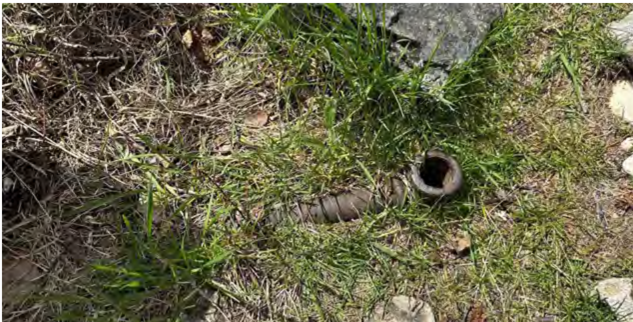
Figure 43: Drainpipe between east stairs of south addition and the south foundation of the main structure of the main lodge.
