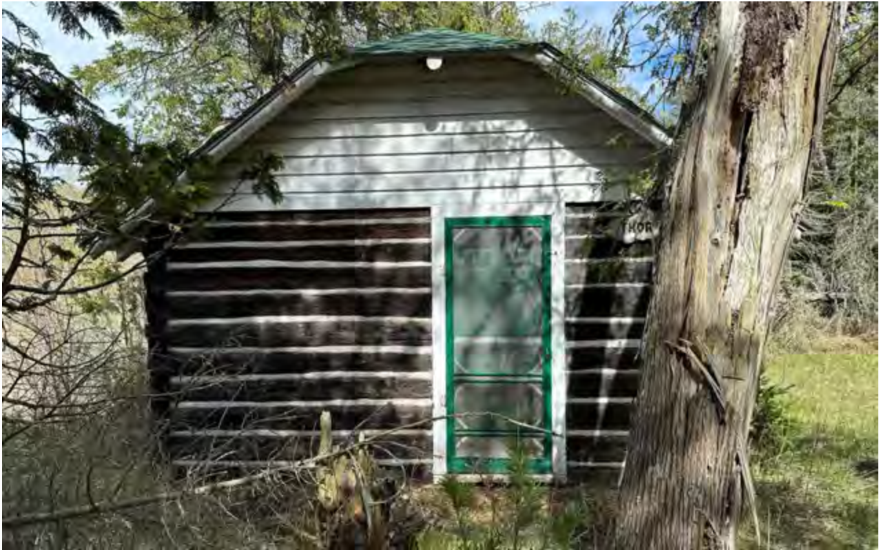
Figure 59: Front/west façade of Thor Cabin, looking east.
