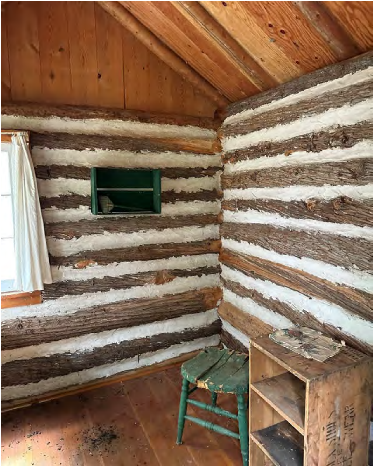
Figure 66: Cupboard and south window in Woodsedge Cabin.
