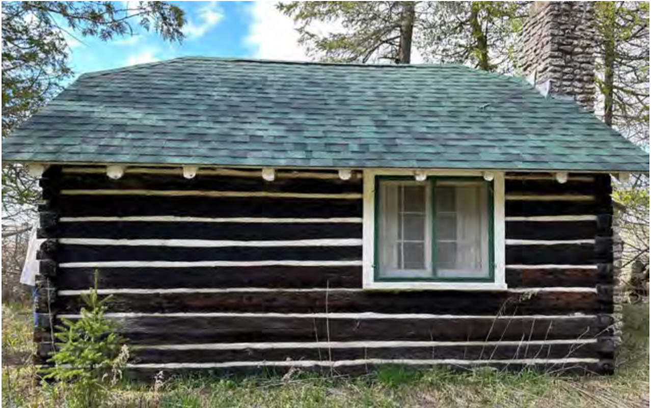
Figure 60: South façade of Thor Cabin, looking north.
