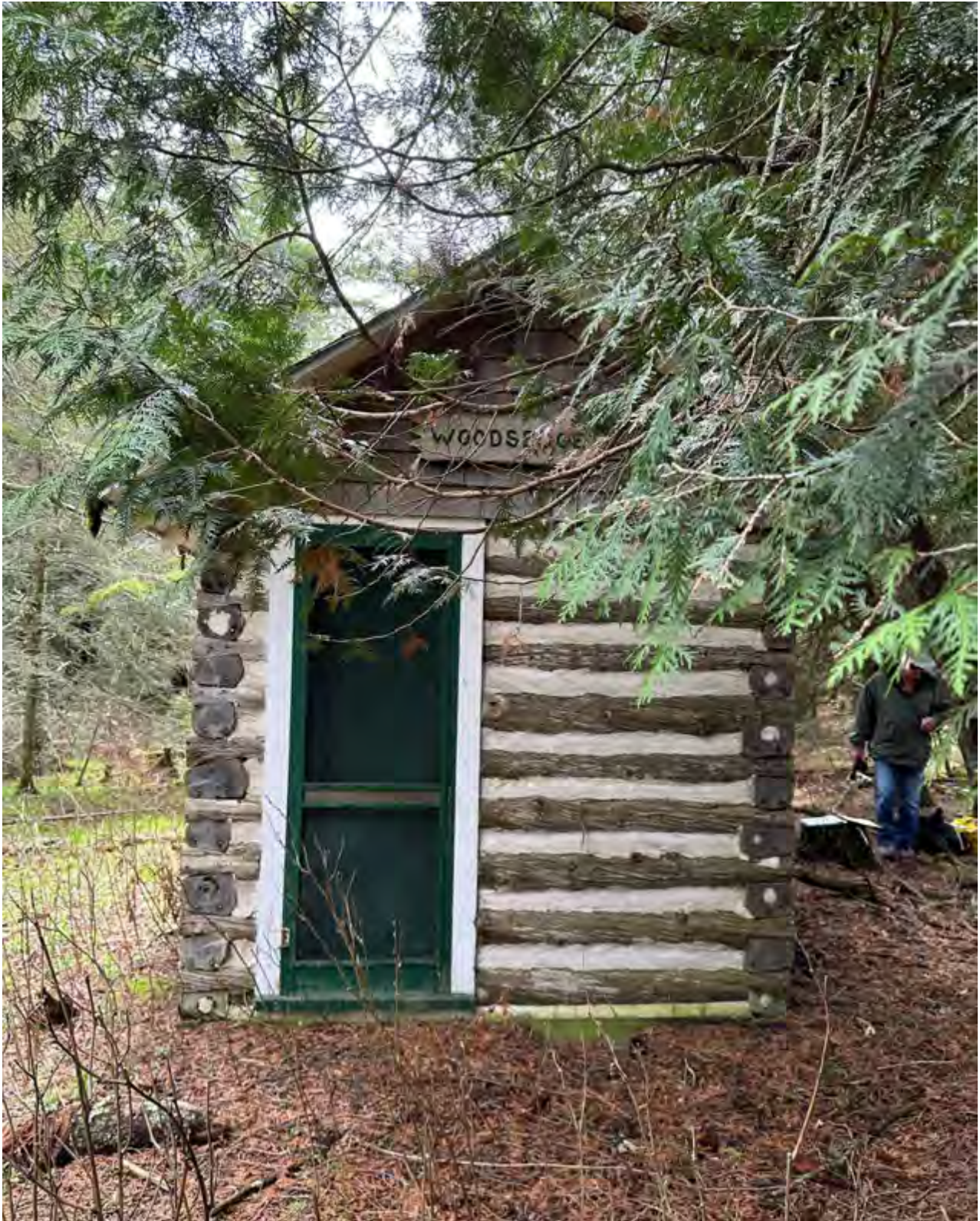
Figure 63: Front façade of Woodsedge Cabin, looking south
