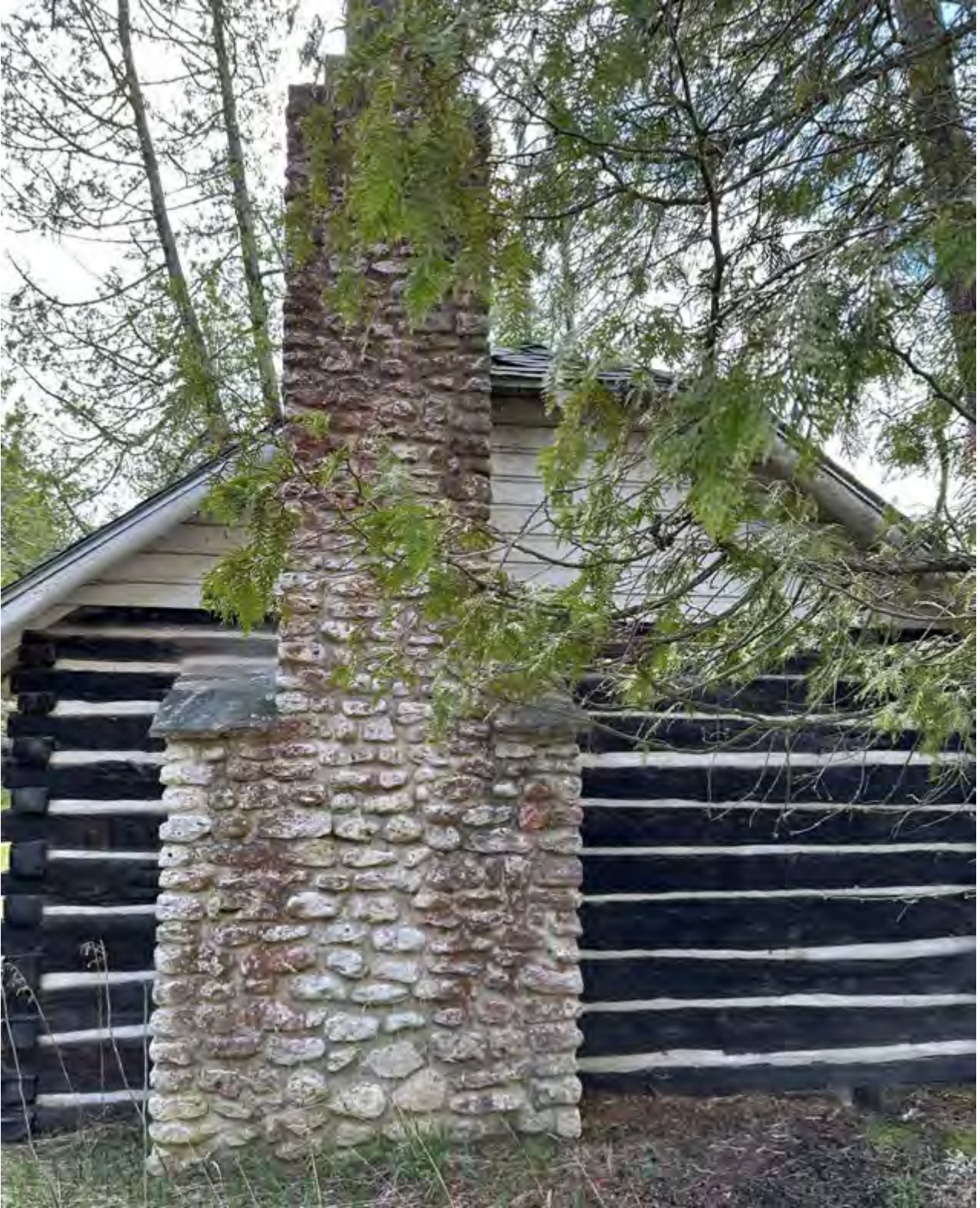
Figure 62: Chimney on east façade of Thor Cabin, looking west.
