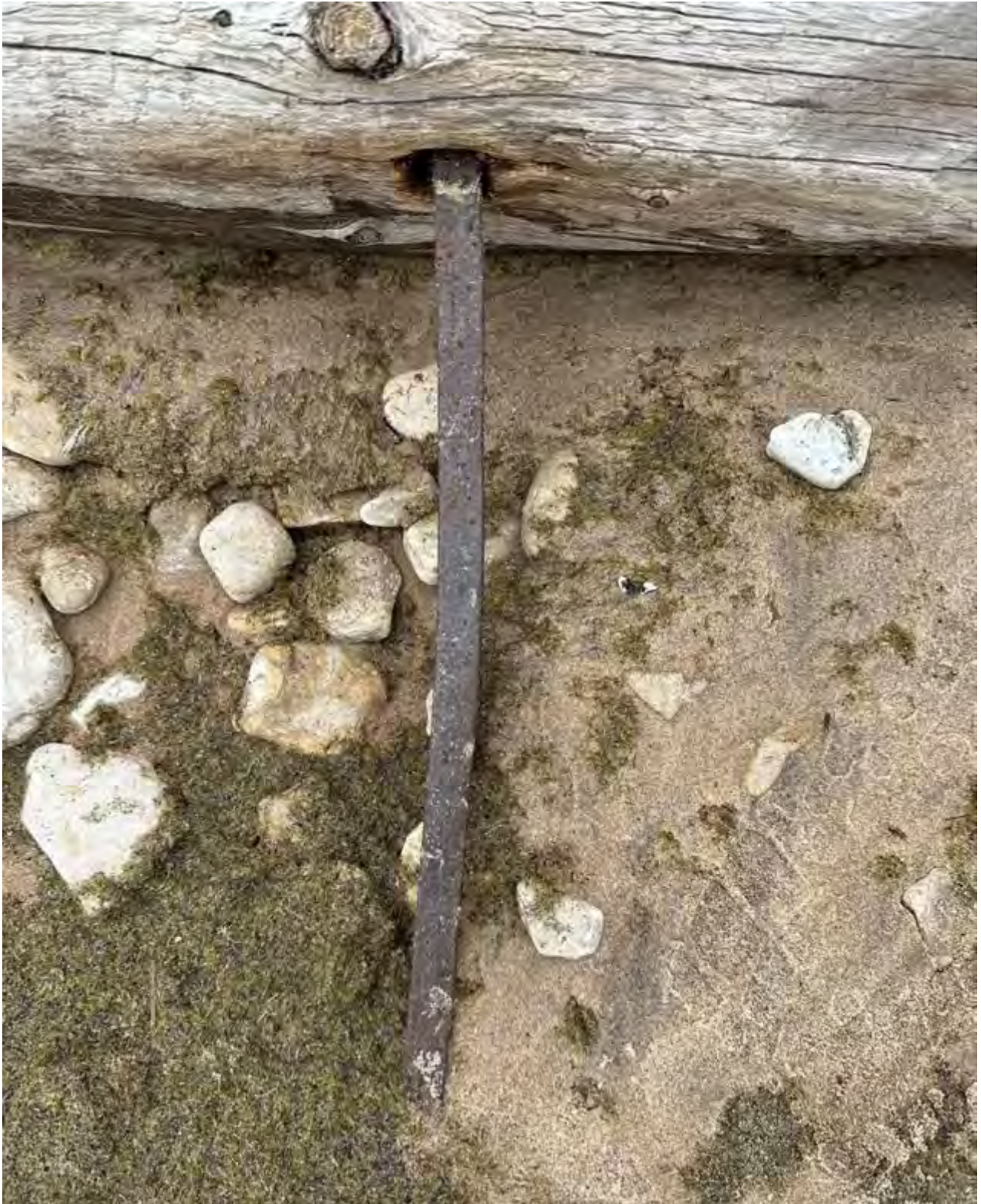
Figure 113: A crib timber with drift pin attached on the beach at Newport.
