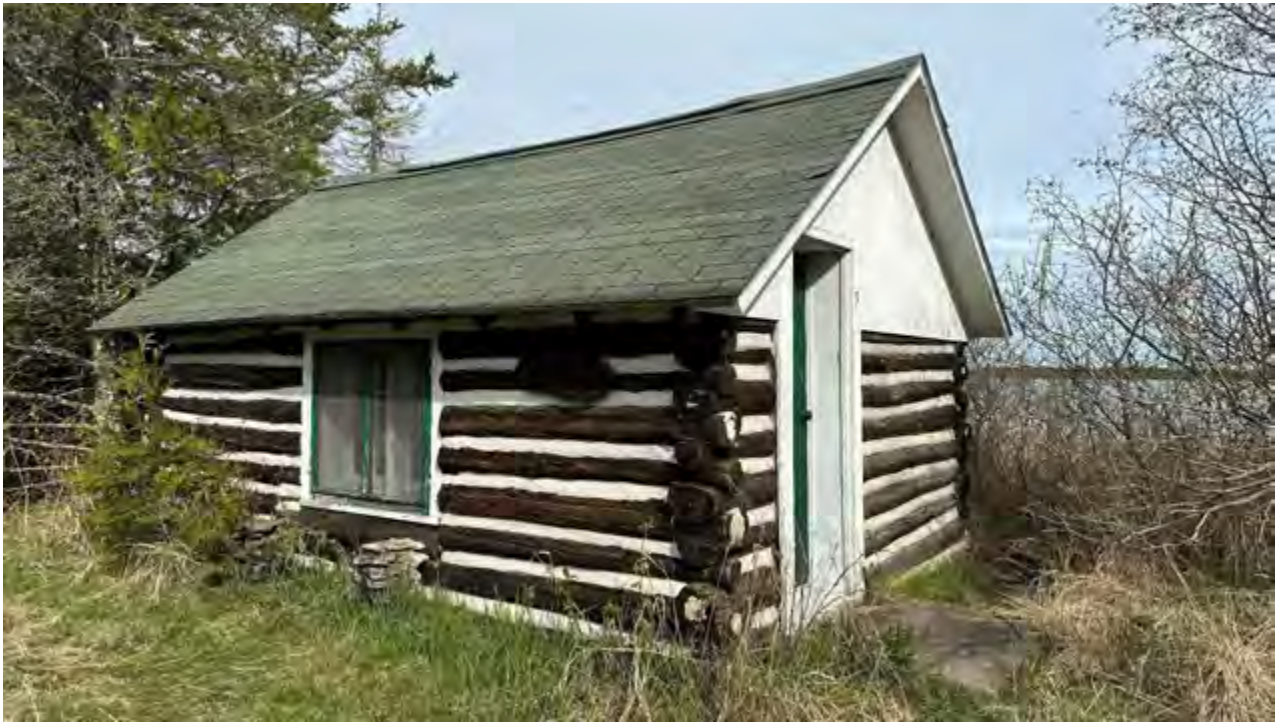
Figure 55: East (right) and south (left) facades of Jeannie Cabin, looking northwest.
