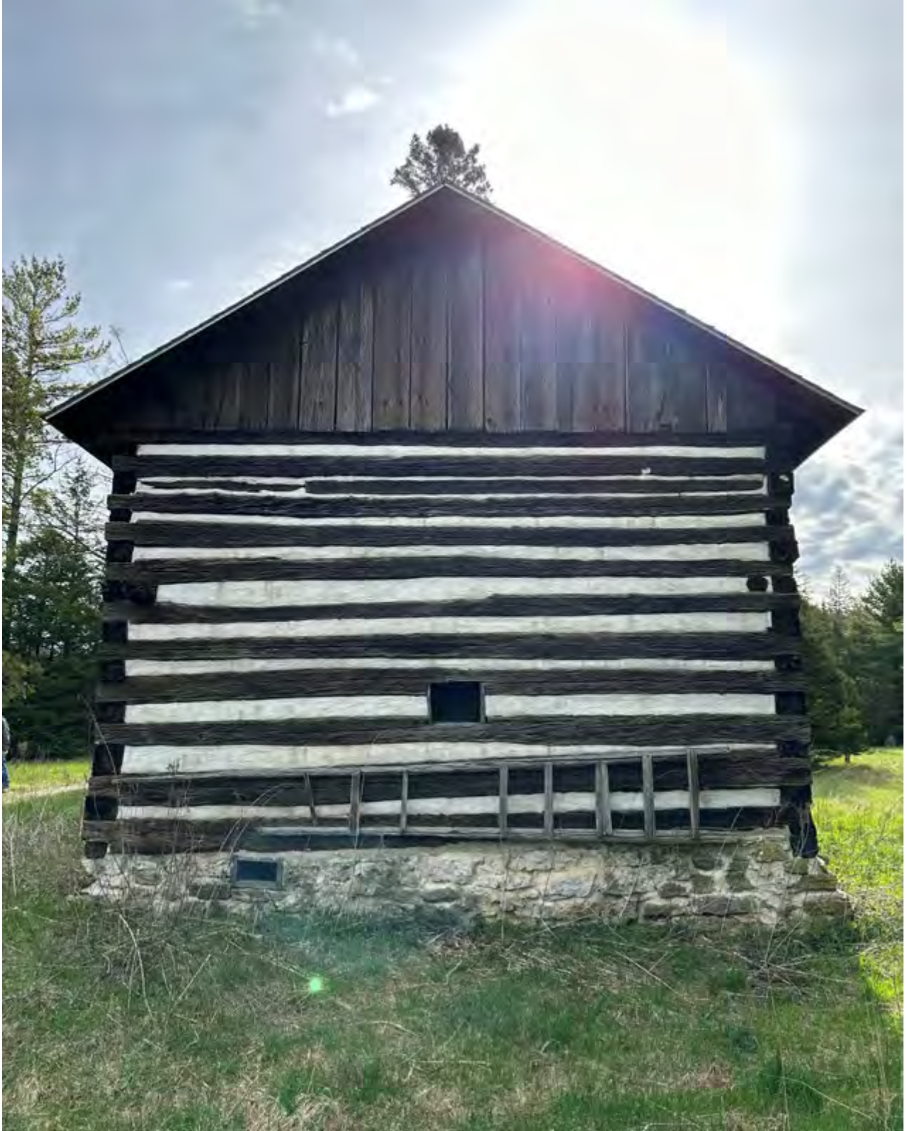
Figure 47: The west façade of the barn at Toft Point, looking east.
