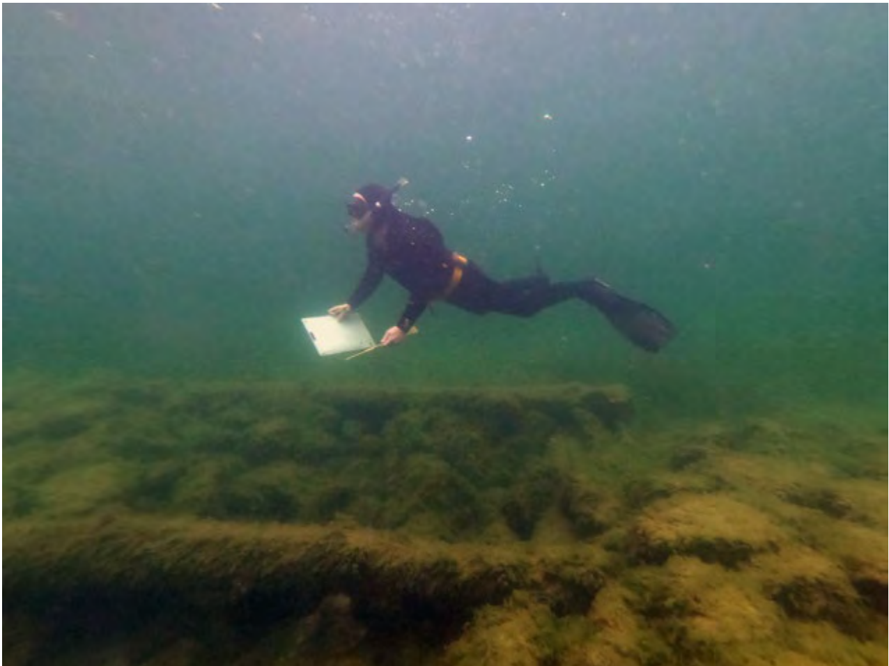
Figure 107: Volunteer Tim Pranke free dives down from the surface to examine Crib 7.
