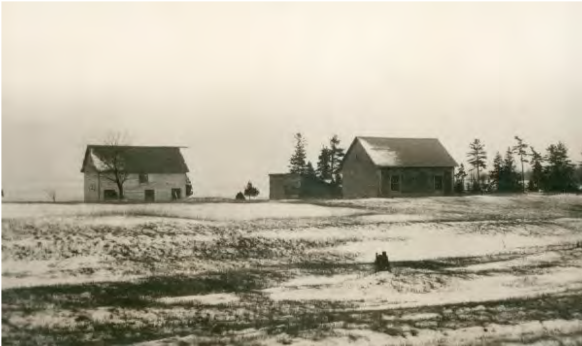
Figure 128: Abandoned outbuildings in the vicinity of GPR Block 5 in 1921, looking southeast. Wisconsin Historic Image 94453, Ferdinand Hotz collection.
