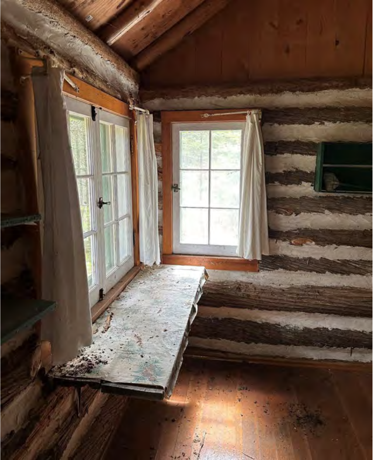
Figure 65: Shelf and east window from interior of Woodsedge Cabin.
