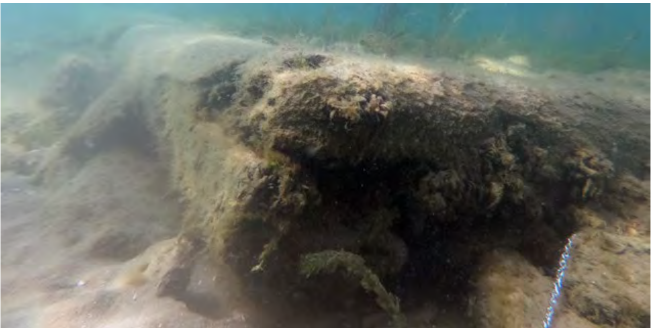
Figure 86: Drift pin-secured corner at Higgins Pier.
