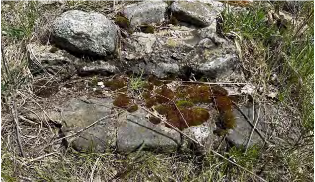
Figure 41: Stairs on east side of southern addition to Main Lodge.
