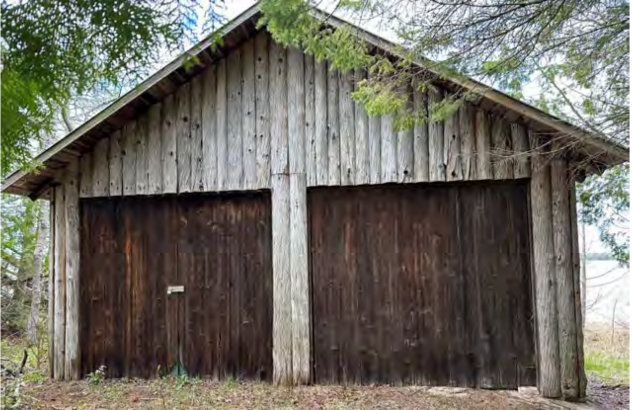
Figure 52: Front façade of Boathouse, looking north.
