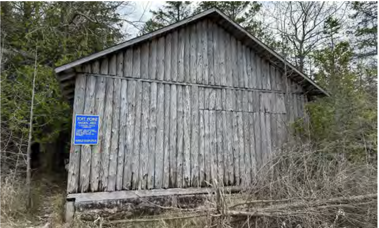
Figure 53: North/rear façade of Boathouse, looking south-southwest.
