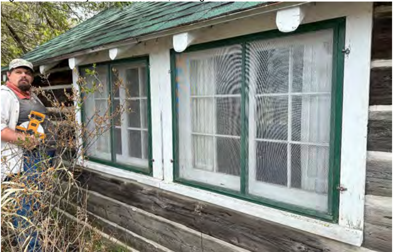
Figure 61: Detail of north façade of Thor Cabin, looking south. Jordan Ciesielczyk to left.
