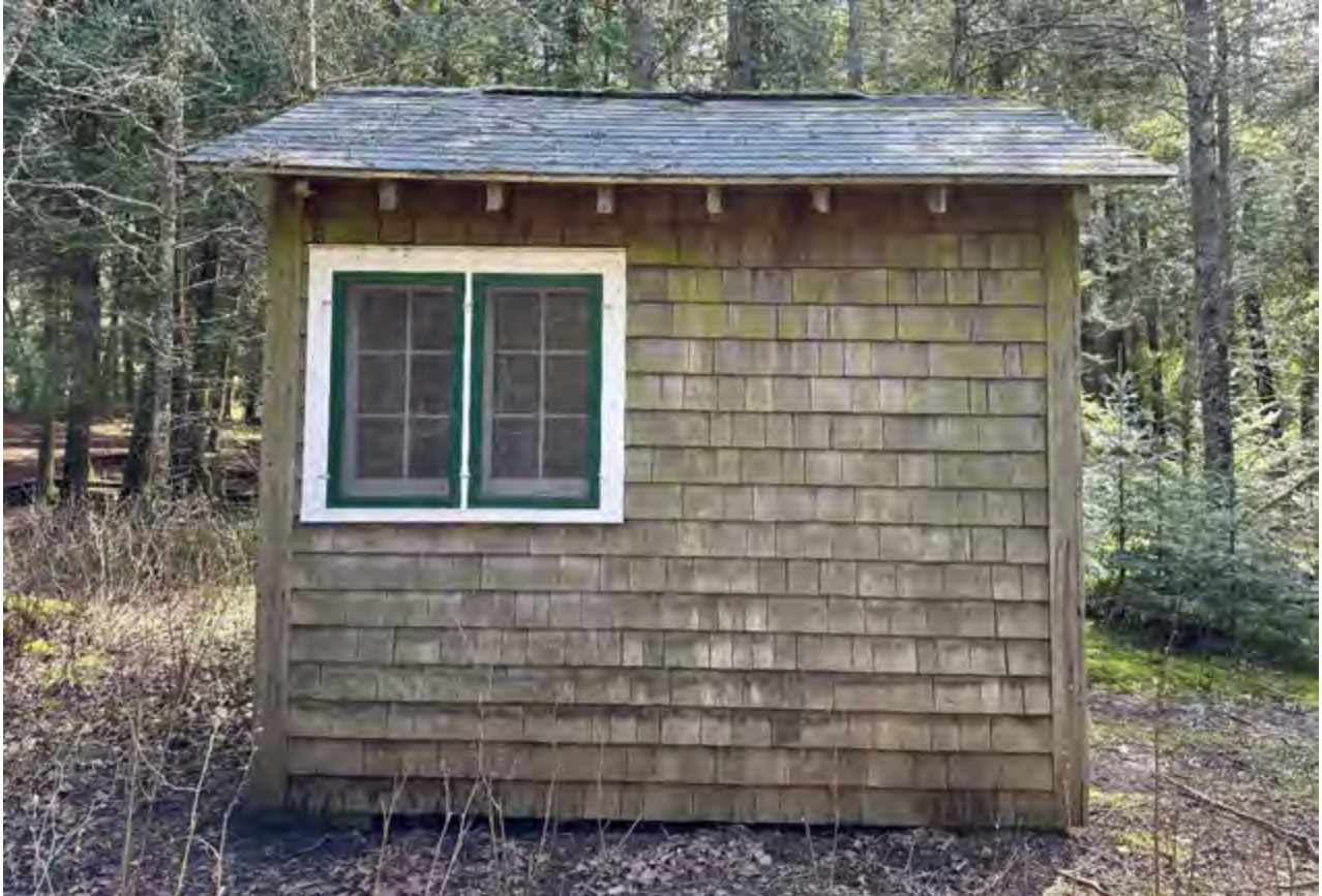
Figure 70: South façade of Fern Cabin, looking north.
