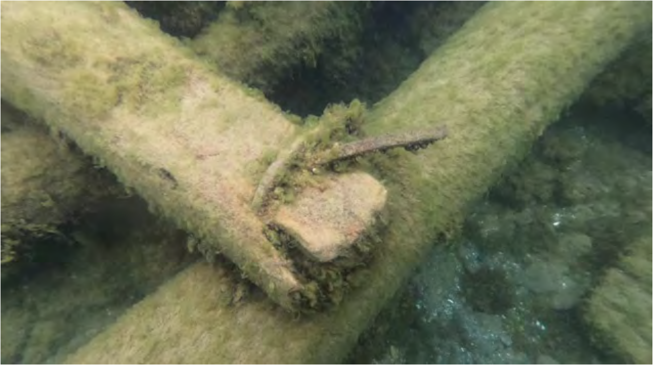
Figure 110: A bent drift-pin connects two crib timbers.
