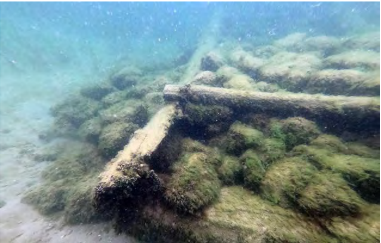
Figure 111: Crib fill spills out from a crib structure.
