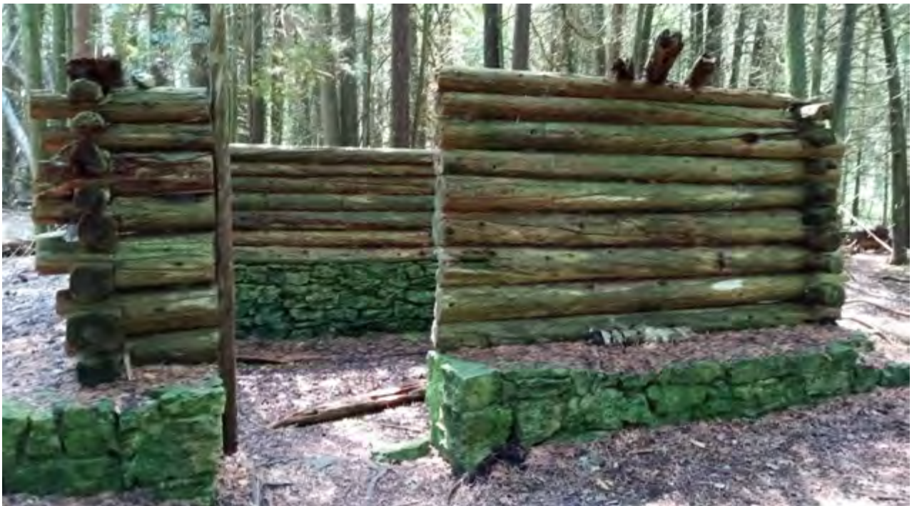
Figure 50: Photograph of the front façade of the icehouse, looking south.
