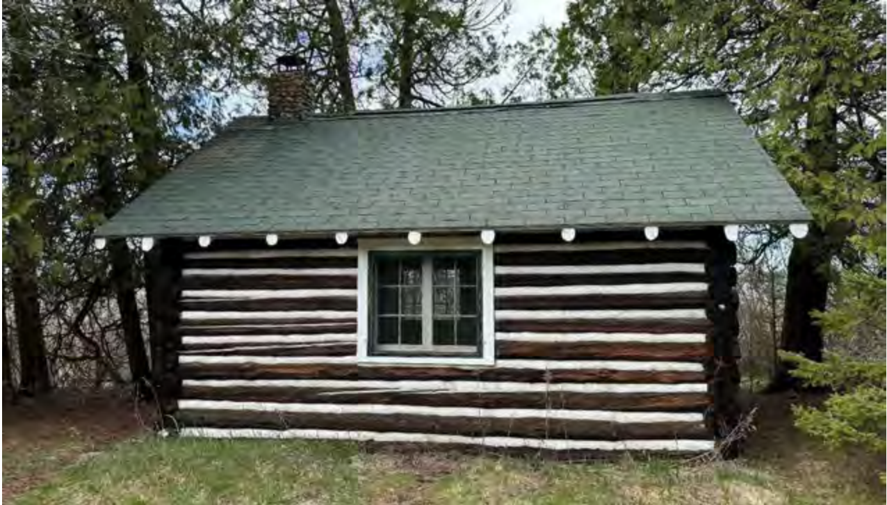
Figure 58: South façade of Juleyanne Cabin, looking north.
