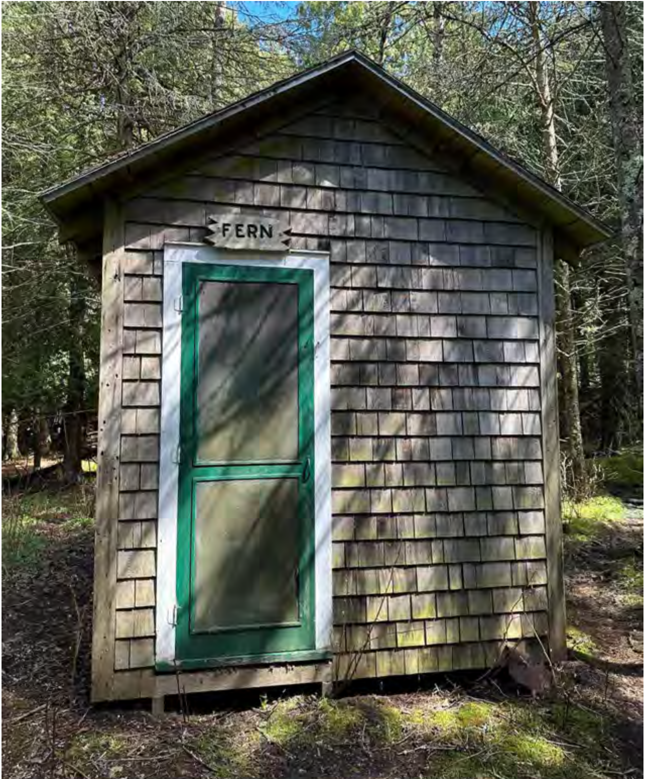
Figure 68: Front/west façade of Fern Cabin, looking east.
