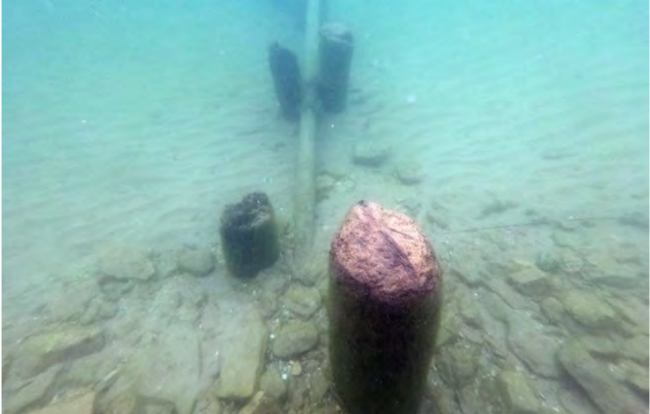
Figure 161: Pilings and a fallen post in the nearshore section at Whitefish Bay.
