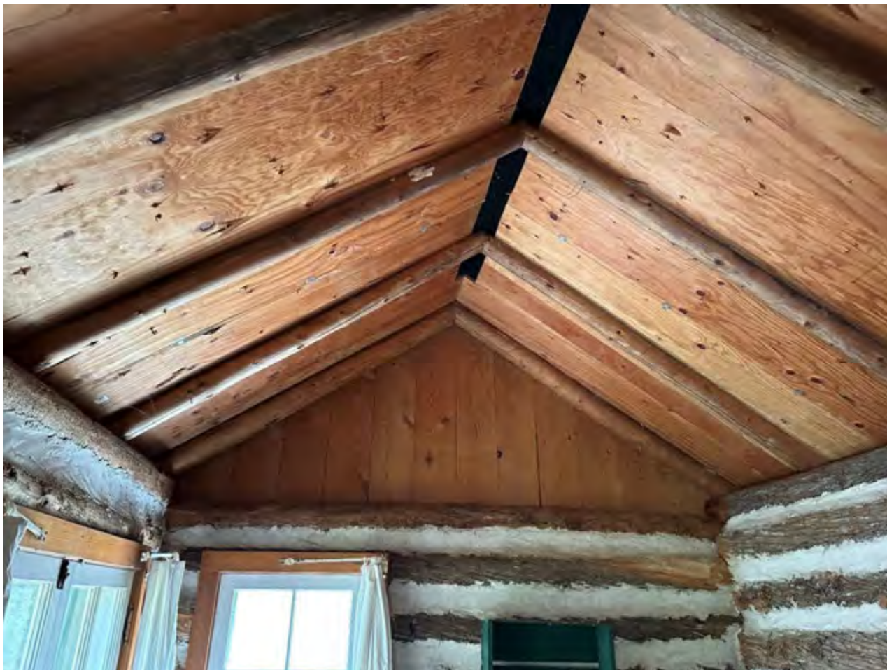
Figure 67: Underside of roof in Woodsedge Cabin.
