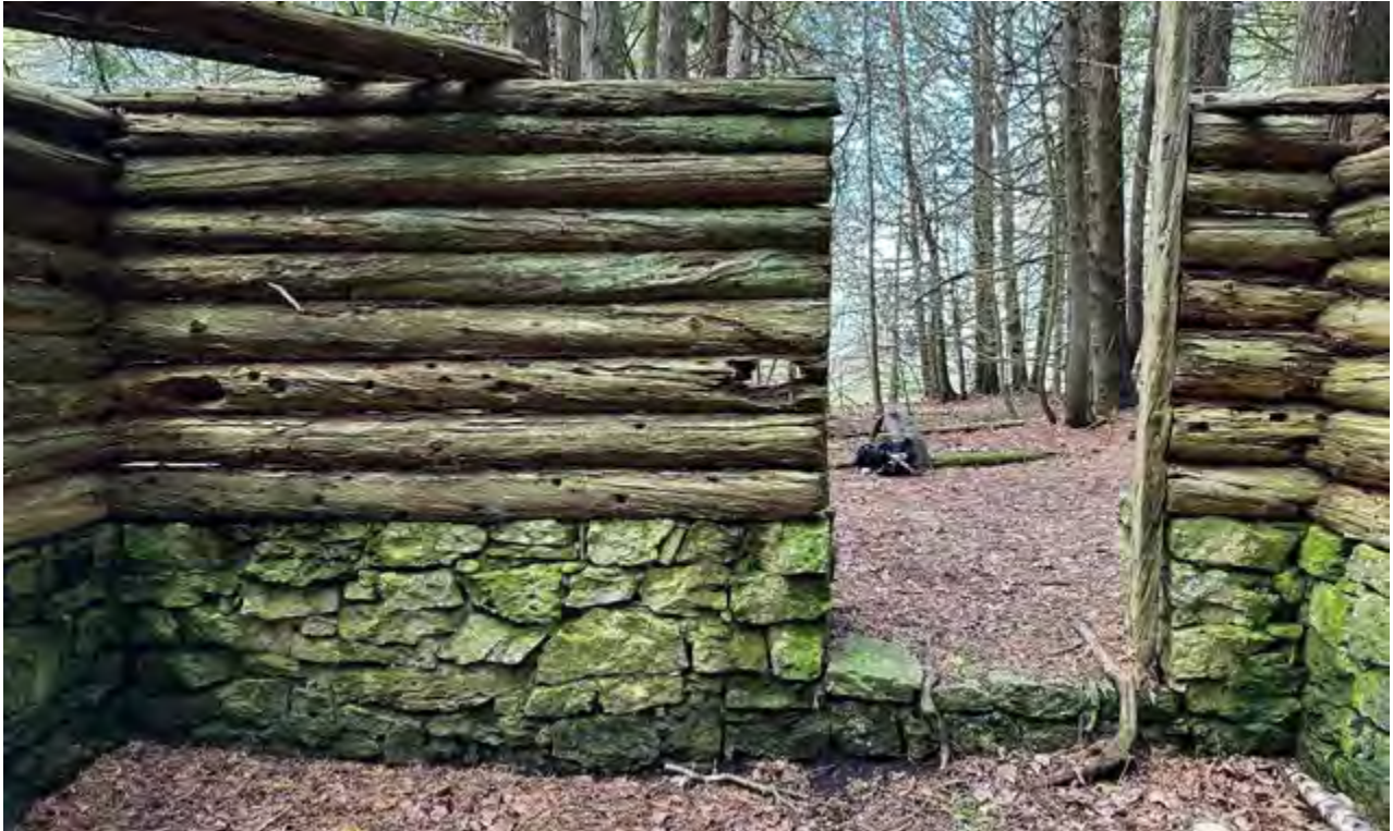
Figure 49: Photograph of the interior foundation of the icehouse, photograph looking north towards entryway.
