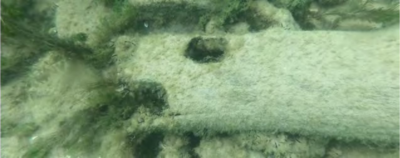
Figure 85: Detail of drift pin in notched crib timber Higgins Pier.
