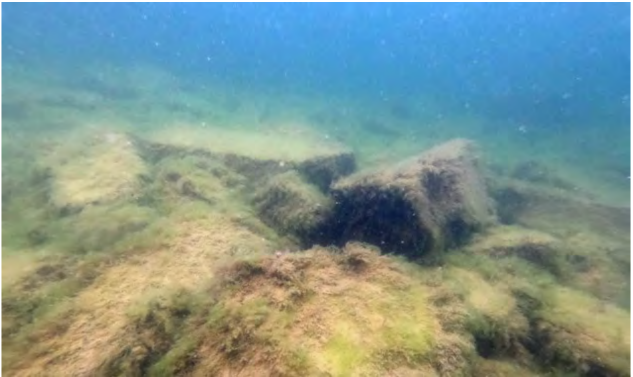
Figure 142: Cribbing stones belonging to Torstenson's pier.
