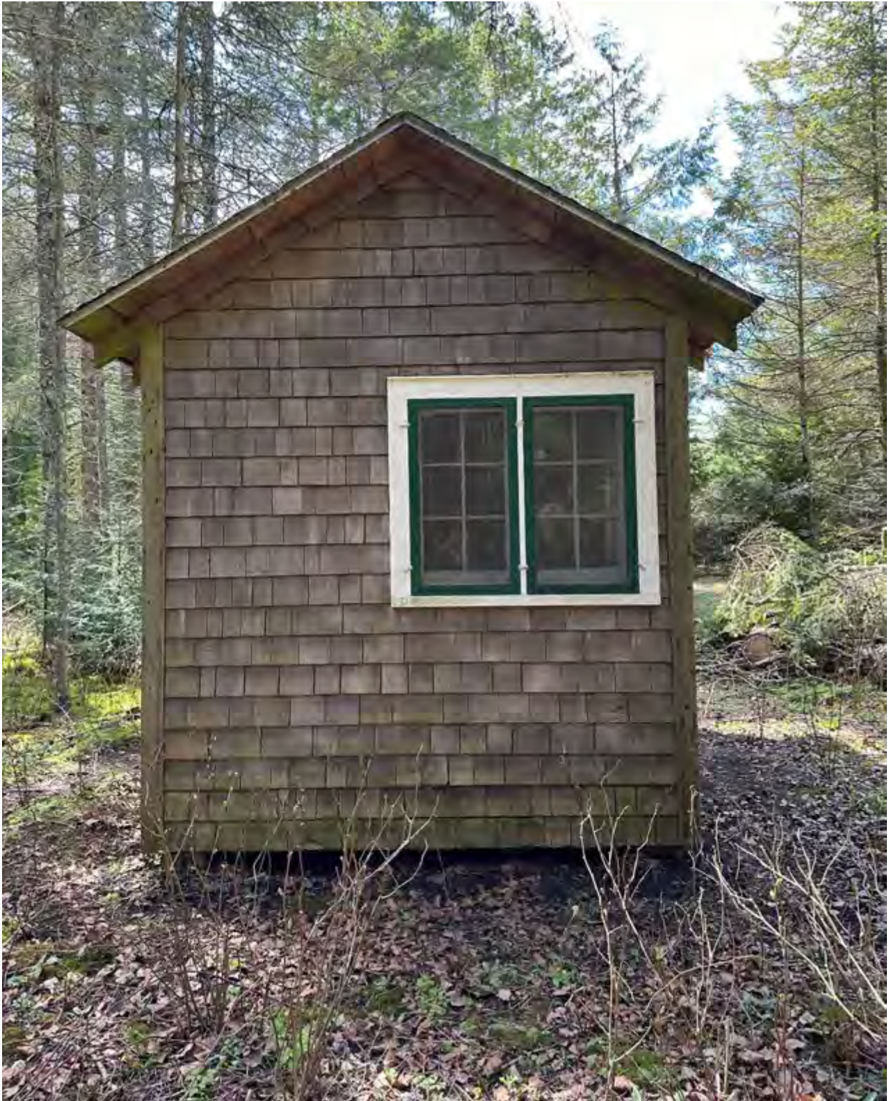
Figure 69: East façade of Fern Cabin, looking west
