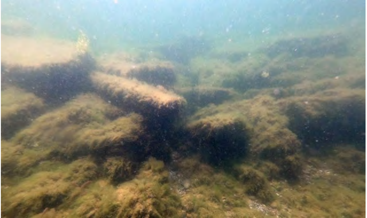
Figure 141: Cribbing timbers and stones from Torstenson's Pier
