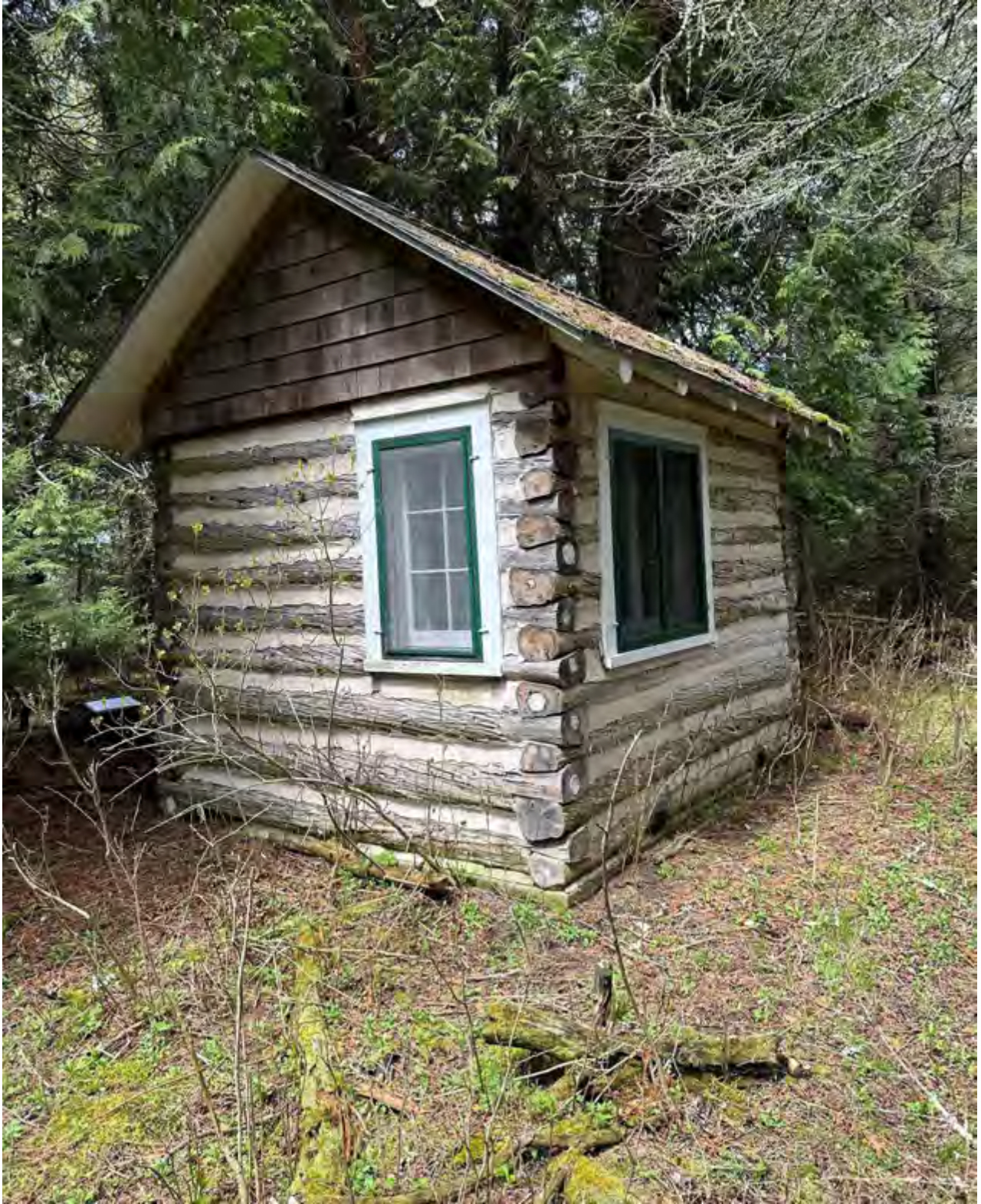
Figure 64: South and east façades of Woodsedge Cabin, looking northwest
