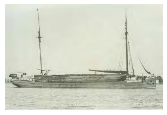
Figure 12. The A.C. Tuxbury loaded with wood. Image taken after her 1905 conversion from three masts to two. University of Michigan Library.
